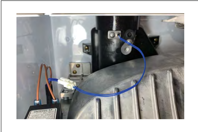
Figure 67 Exhaust Temp. Sensor
