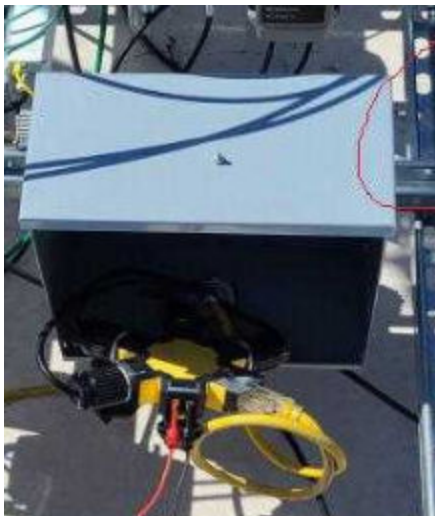
Multiple grounding wires connected to a single point
