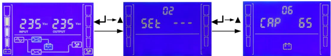
Figure 5-5 Setting the battery capacity
