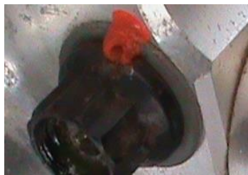
Figure 13 - Torque seal installed
