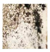
Mould can be mostly found in houses with rising damp and poorly ventilated areas, such as bathrooms or built-in wardrobes. Good ventilation and decreasing humidity are key to tackling mould issues.
