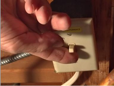
• Once the new filter is installed, find the power switch again and flick the switch to the "on" position.
