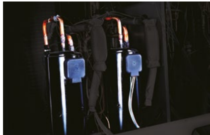
Multiple large-capacity all inverter compressors (from 14 HP).
