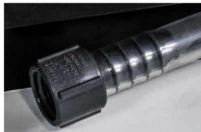
DRAIN TUBE bottom front of cooler (condensor side) and connects directly to floor drain
