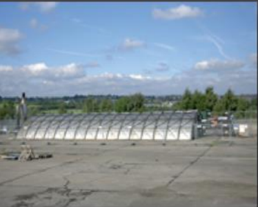
SIDE VIEW OF BURNERS ATTACHED TO CELL
