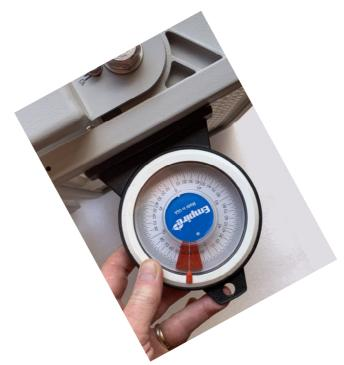
10. Tighten M20 side bolts to 220 Nm so floodlight will no longer move, and confirm installed tilt. Tighten M10 locking grub screw to 40Nm.
