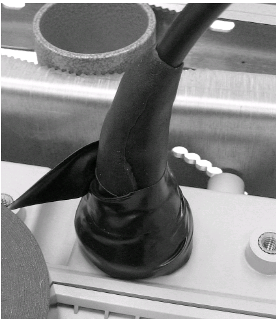
Figure 35 Electrical tape application around the Butyl Rubber
