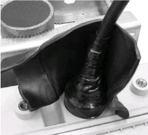
Figure 34 Butyl rubber application
