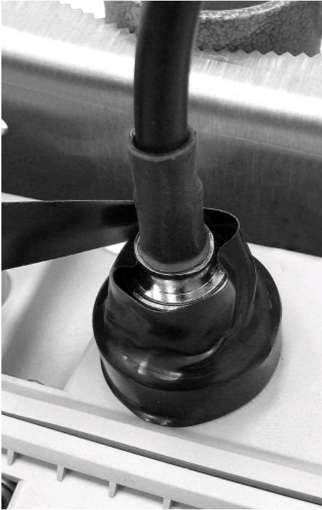
Figure 32 Starting the electrical tape application
