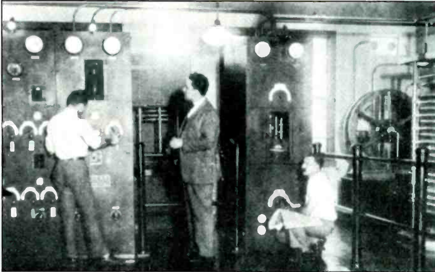
In late 1928, many American broadcasters were forced to shift frequencies. Here's the auspicious occasion of the 50 kW WEAF transmitter actually being retuned from 610 to 660 kHz.
