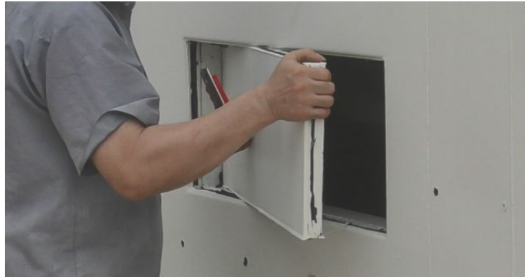
Figure 6-7 Removing the connection box cover
