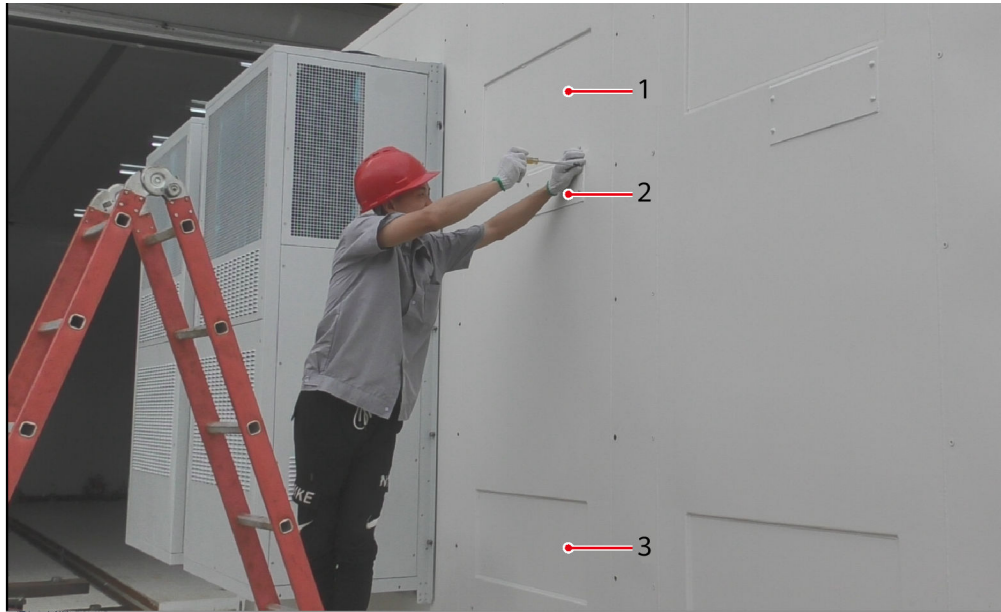
(1) Supply air vent cover (2) Cable connection box cover (3) Return air vent cover
