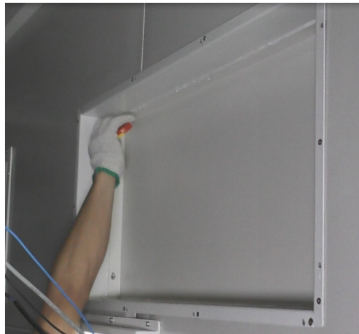
Figure 6-6 Cutting the glue
