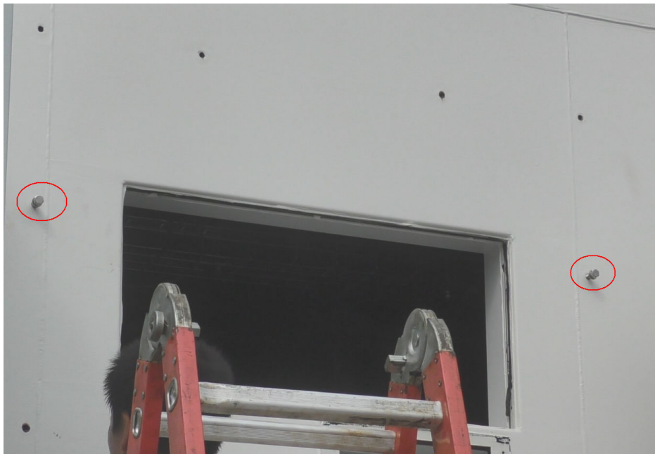
Figure 6-8 Installing two bolts
