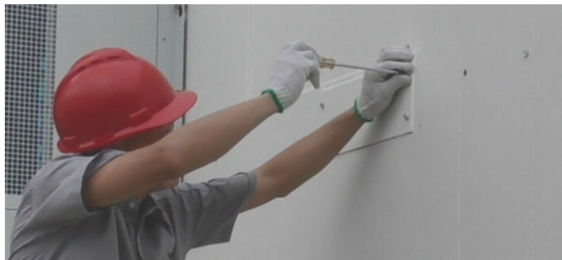
Figure 6-3 Removing the screws on the cover of the connection box
