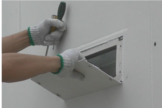
Figure 6-5 Removing the connection box cover
