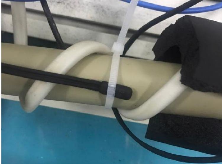
Figure 6-22 Secure the temperature probe
