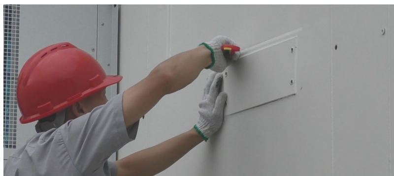
Figure 6-4 Cutting the glue
