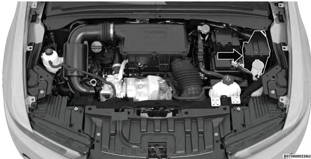
Underhood Power Distribution Location
