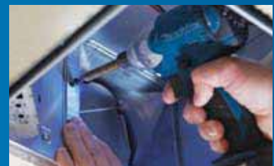
For room-side installation, pull the duct through the opening, attach the duct to the connector, push the connector into place and fasten to the housing with only one screw.
