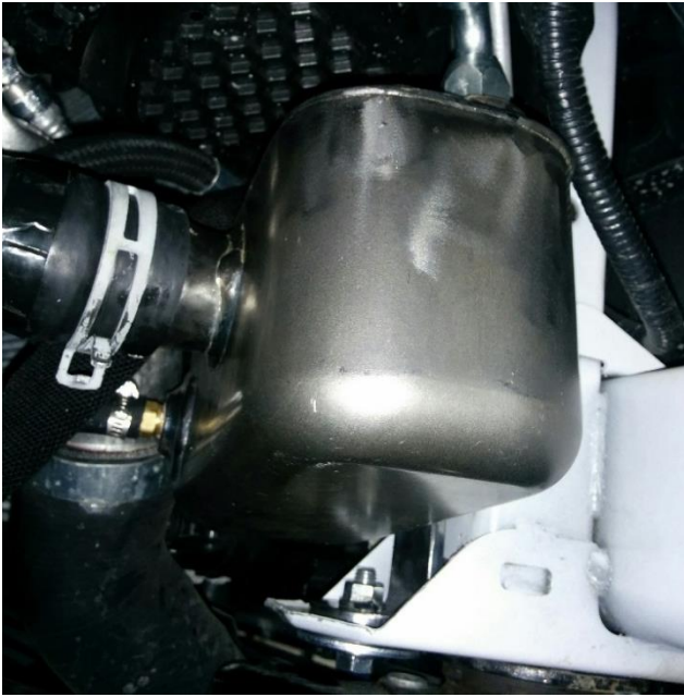
Figure 28 – Installing the cooler
