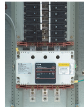
In this installation, the SPD Series is mounted directly to the panelboard’s bus bars. This type of installation will provide the best possible surge protection by minimizing the connected lead length.
