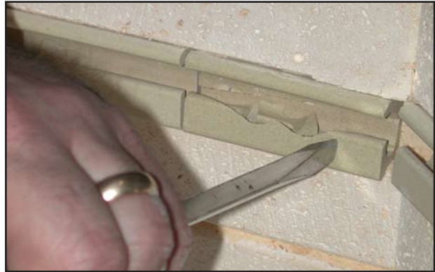
The holder shown with about half the job done:
