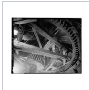
Interior view, Pantigo windmill, East Hampton, New York Historic American Buildings Survey
