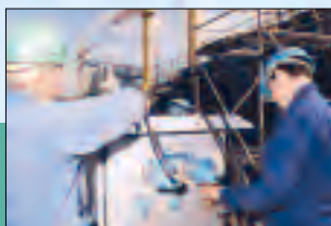
Supply to building sites (shipyards)
