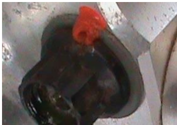
Figure 13 - Torque seal installed
